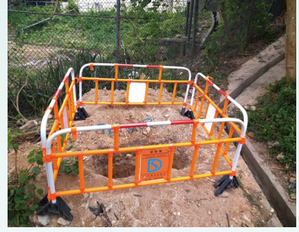
探井挖掘 Trial Pit Excavation
