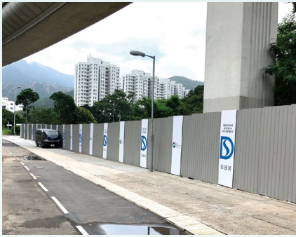
圍板安裝 Hoarding Erection
