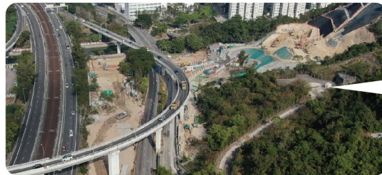
臨時行車天橋地基工程 Temporary Vehicular Bridge Foundation Works
