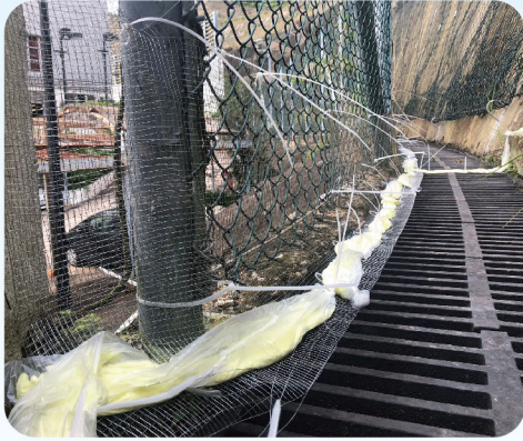
加裝防蛇網及使用硫磺粉 Retrofitted the fences and placing sulphur powder
