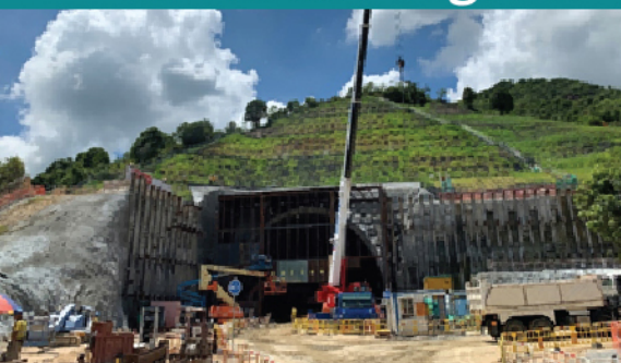
建造主連接隧道 Construction of Main Access Tunnel
