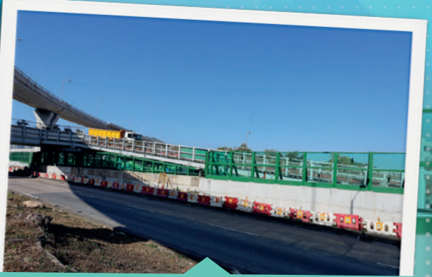
亞公角街臨時隔音屏障建造工程 Construction of Temporary Noise Barriers along A Kung Kok Street
