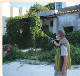
村長表示不少村屋已經塌下荒廢 Many village houses were broken down
